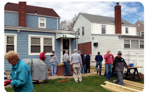
RTLTI volunteers installing a ramp in Mineola
